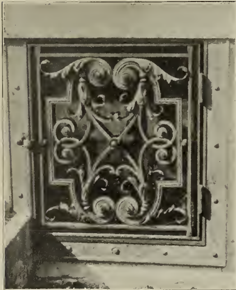
B.—GRILLE FOR BASEMENT. Wrought Iron.
